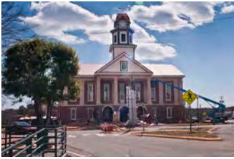
Chatham County 1881 Courthouse reconstruction (Photo by Ava Barlow)
